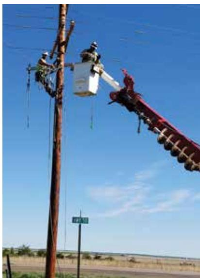
**Left: Linemen climb a pole and utilize a bucket truck to complete repairs on a section of line.**
